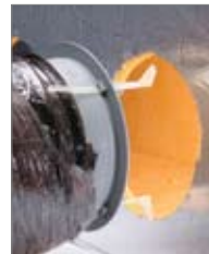
Duct Board Trunkline
