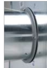
Sheet Metal Trunkline
